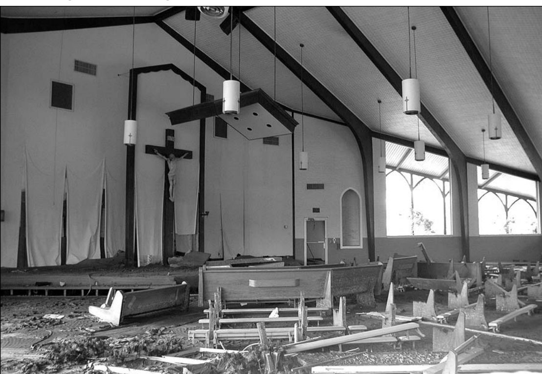
The wind, rain and storm surge removed most of the pews and other furnishings from Our Lady Star of the Sea in Cameron.
